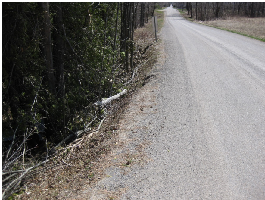
Photo 5B - Narrow Platform Width
