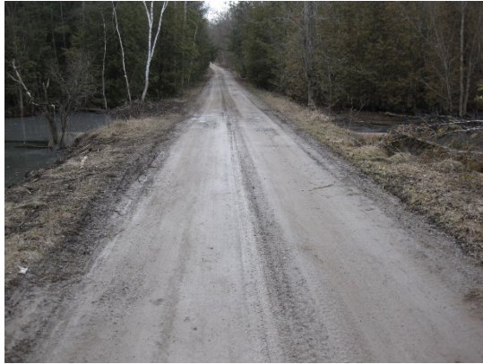
Photo 5 & 5A- Narrow Surface and Platform Widths
