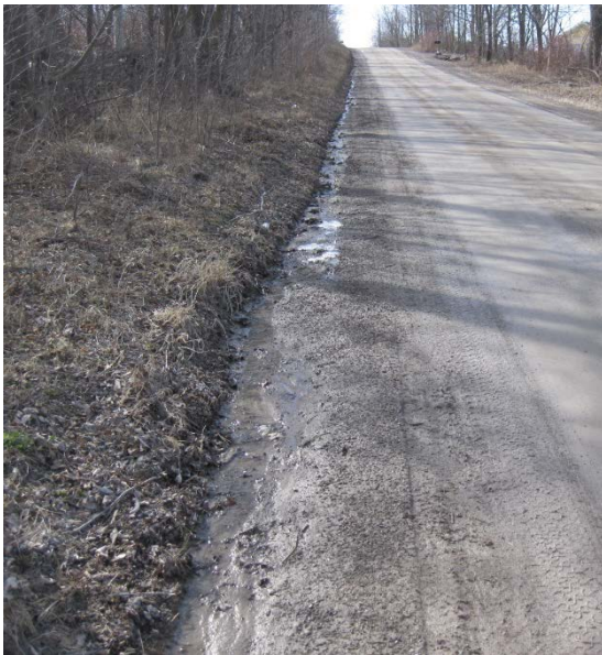
Photo 4&4A - High Shoulders Preventing Surface Water Runoff
